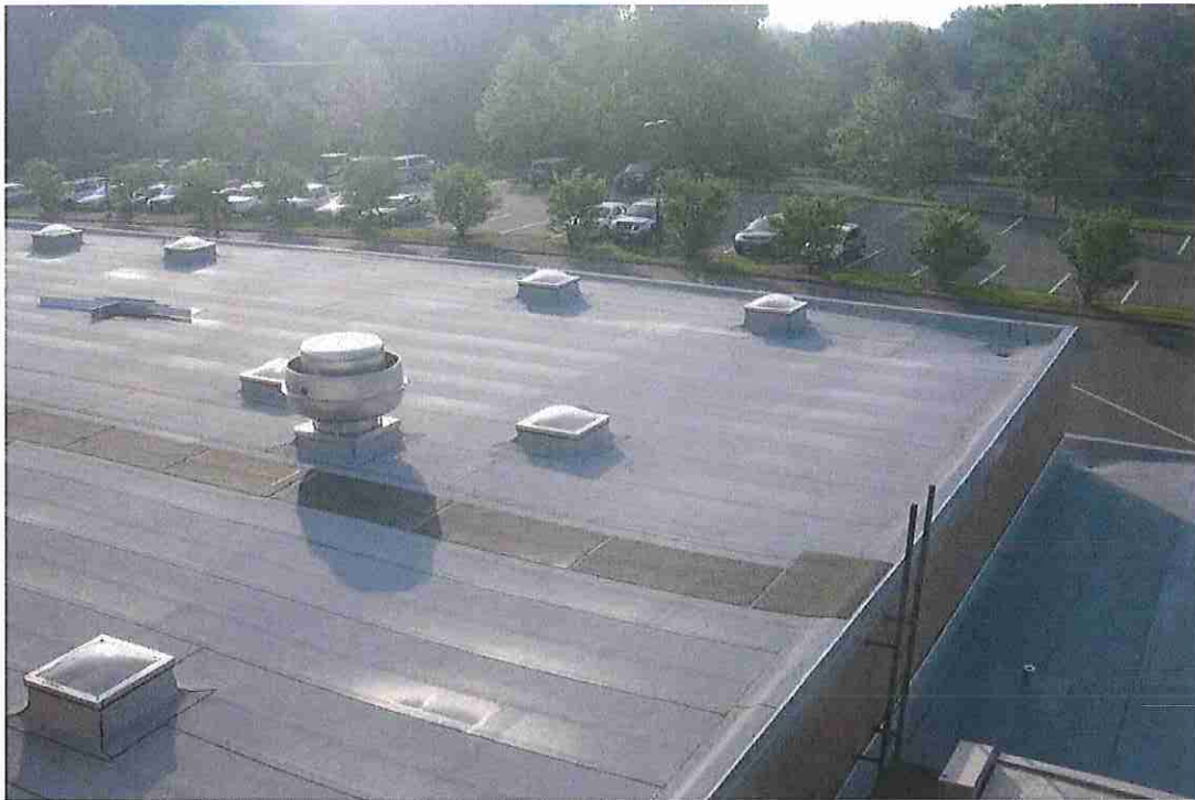
New 2013 roof system at Fairfield Warde High School
