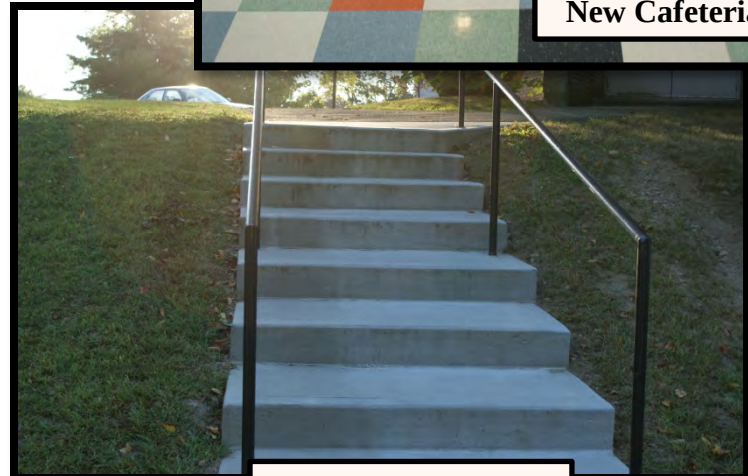
New Concrete Stairs
