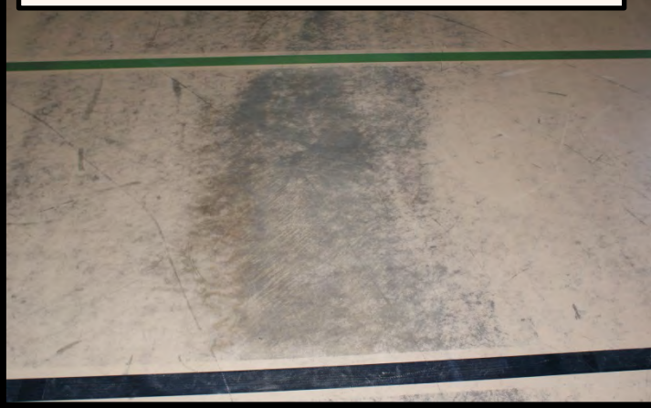
Old Gymnasium Rubber Floor “No Sealer”
